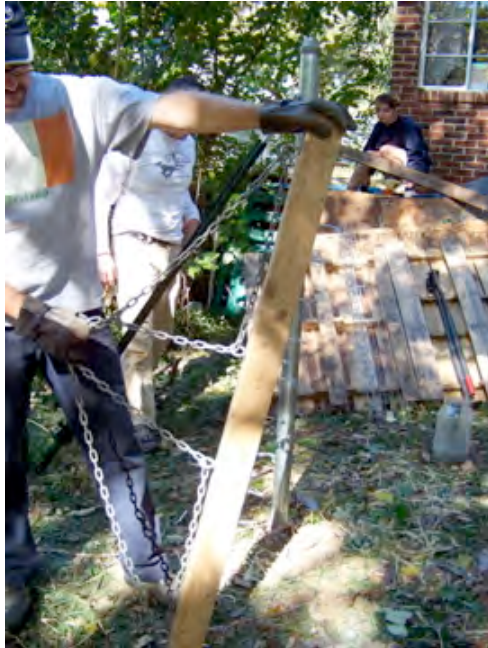
Figure 21. Fence puller (a.k.a “the CUD”)
