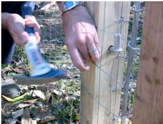
Figures 18 & 19. Staple welded wire to corner post
