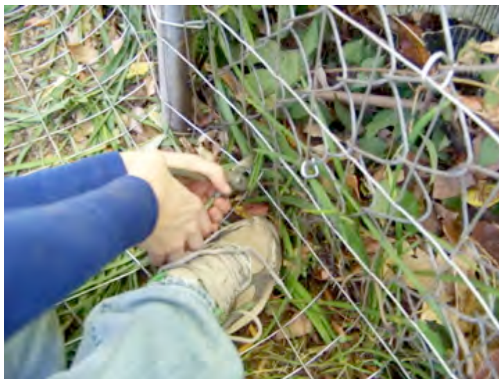
Figure 40. Attaching the ground wire to the fence
