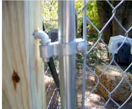
Figure 35. Top lag screw with hinge
