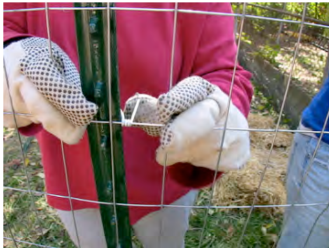
Figure 26b: Soft tying the welded wire to t-post
