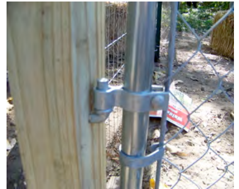
Figure 36. Bottom lag screw with hinge
