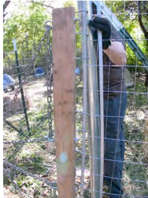
Figure 22. Attach fence-puller to tension bar
