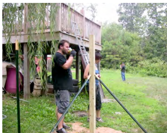
Figures 6a and 6b. Placement of the diagonal supports against vertical t-posts
