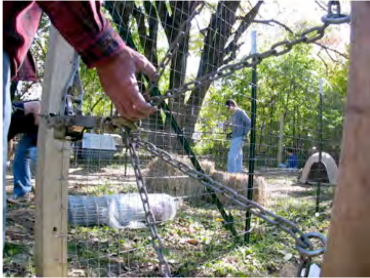
Figure 24. Attach the come-along to the fence puller
