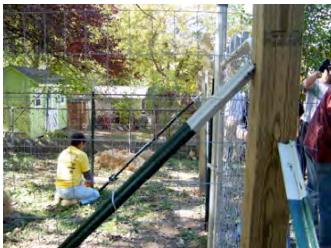
Figure 5. Placement of diagonal support
