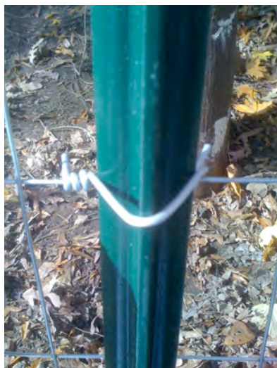
Figure 26c: Soft tie holding welded wire to t-post
