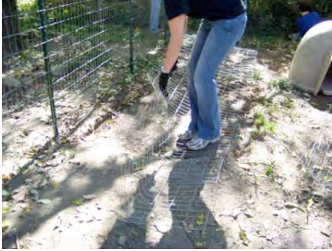
Figure 38. Fold the welded wire along the fence.
