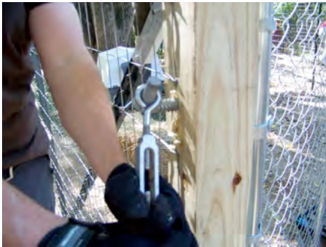
Figure 34. Screw in the lag screws
