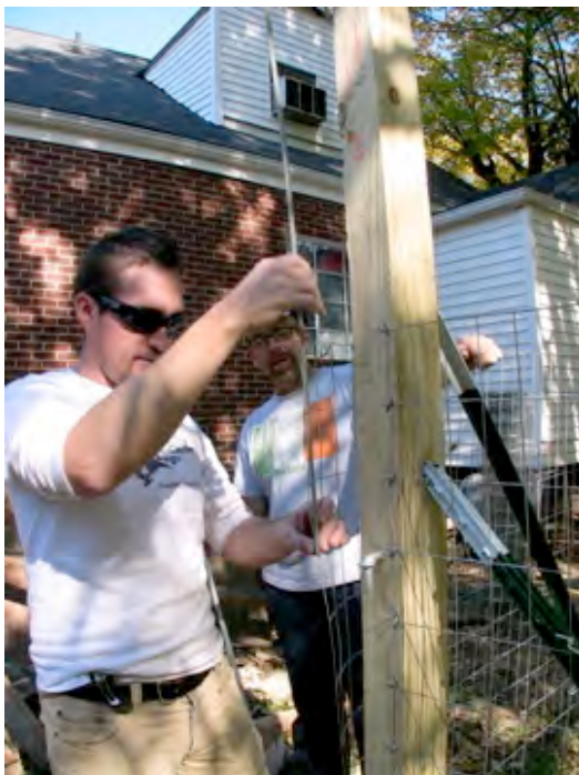
Figure 20. Weaving the tension bar through the welded wire
